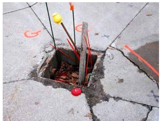
Those of you who never frequent these streets may not know how badly they have deteriorated.
